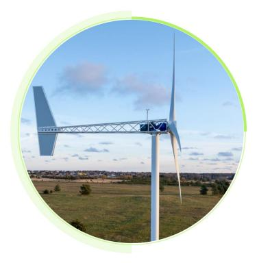
The main parts of the wind turbine are foundation, tower and nacelle with rotor and tail, electric panels and cables necessary for energy transfer and turbine control. Wind turbine has free yaw with tail. The turbine rotation speed is constant. For safe operation blade tip-brakes will activate with rotor over speed and mechanical rotor brake is used to stop the rotor. All these methods allow for safe operation and control of the turbine.
